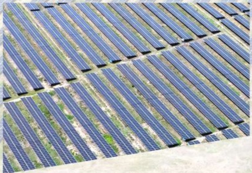
SPACE TEXTILES - TIRUPPUR CAPACITY-3.6 MW
